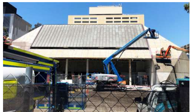
Sir John Clancy Auditorium undergoing foyer renovations
